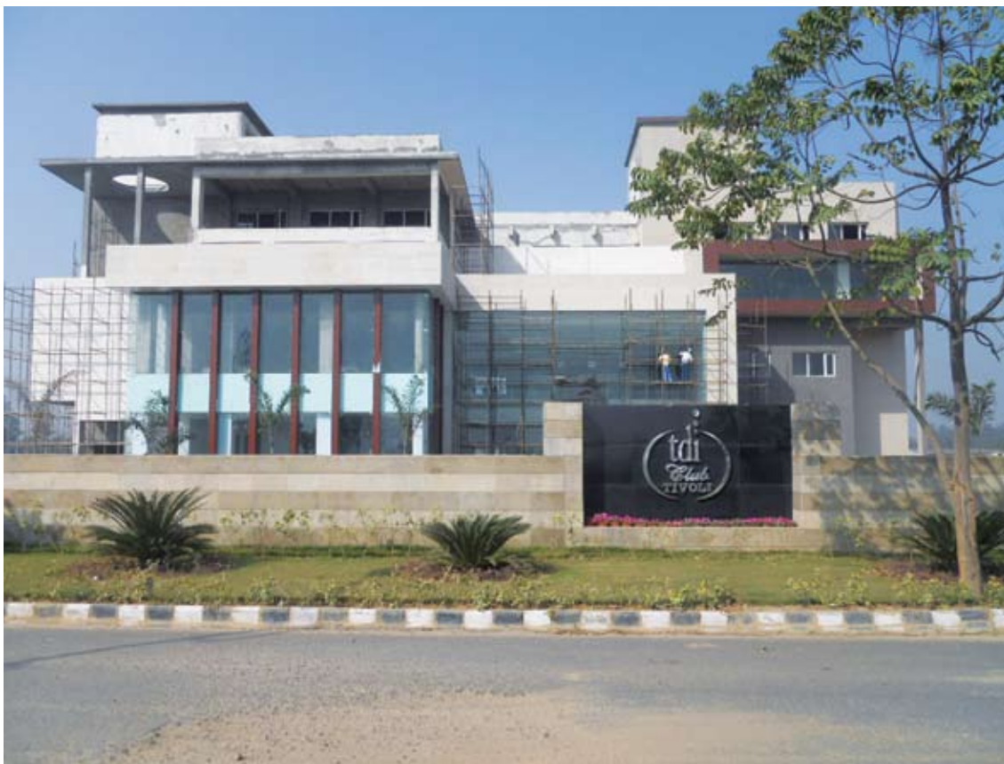
TDI Club, Tivoli: An opulent recreational club in Block- A, Phase-I soon to be operational. Conference hall and Coffee Shop ready and work is on at the front park and parking
