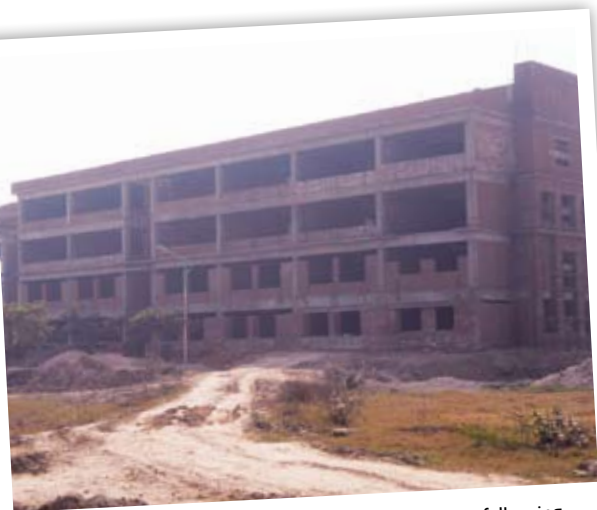
TDI International School in E-Block; construction in full swing
