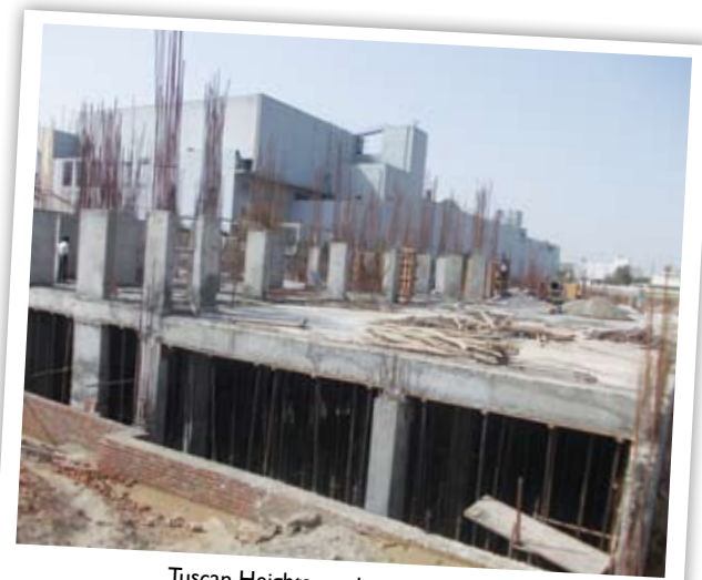
Tuscan Heights- under construction
