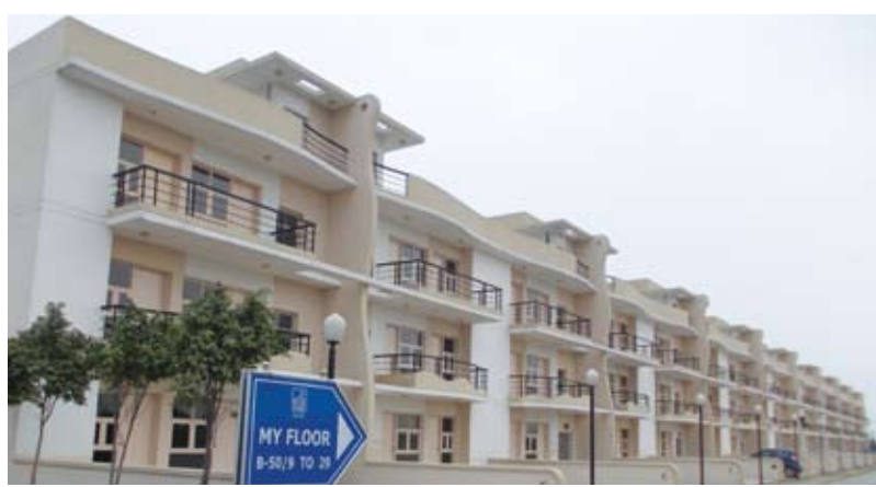
My Floors-I: Possession handed over; many have moved in and more in the process of moving in.
